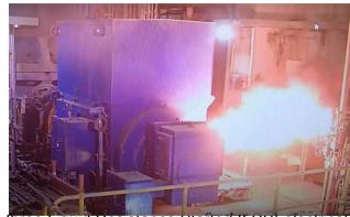
The incident was caused when two of the three Liquid Resistance Started (LRS) electrical phases (red & white) came into contact resulting in short-circuit and thus created a spark that ignited the carbon filings/build up. This resulted in the arc flash/blast during the restart process of CR01.
