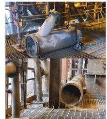
There were a lack of pipe supports in the pipeline and several existing pipe supports had failed through corrosion. The pipeline had additional weight due to the accumulation of settled process solids.
