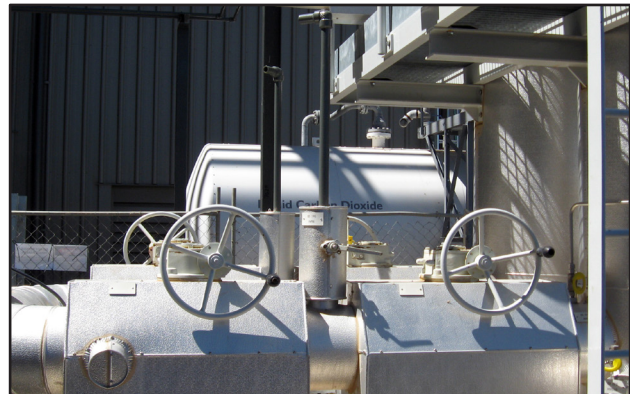
Typical Double Block and Bleed
