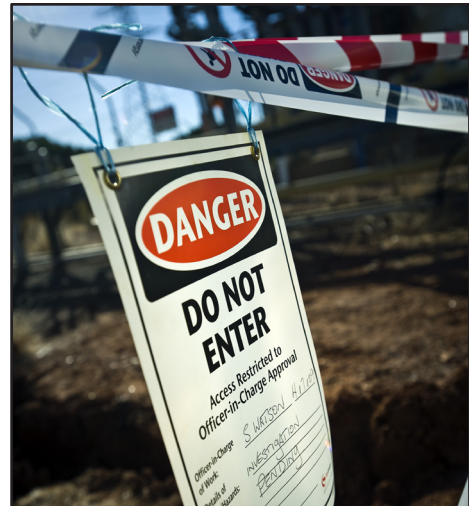
Danger Sign and Barricade
