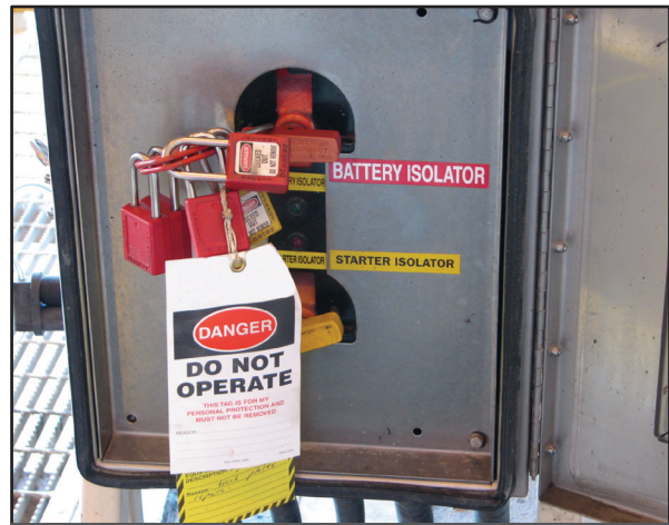
Typical Mobile Equipment Isolation Point
